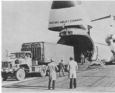
At McGuire AFB, DAS3 was certified for loading aboard the CSA and C141.
